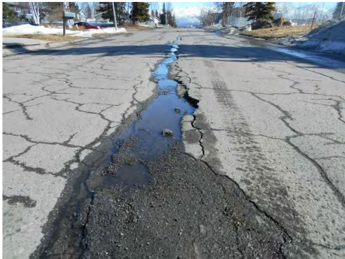
Drainage and ponding issues on 48th Avenue, shown here, need to be repaired.
