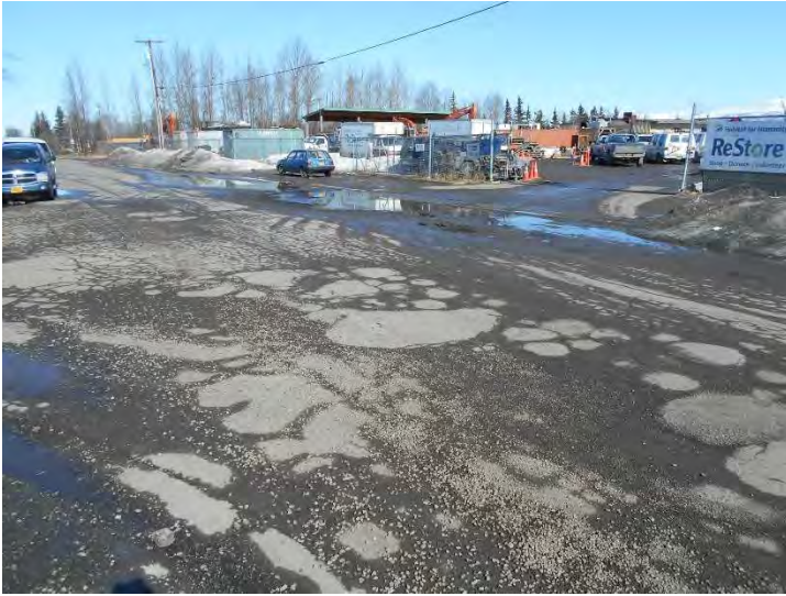
Poor asphalt conditions and roadway ponding are observed on Cordova Street.
