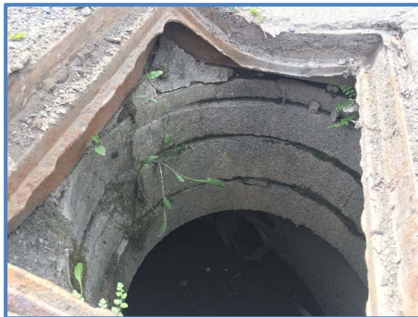
Photo 3 - Frame, Grade Rings & Reducing Slab
