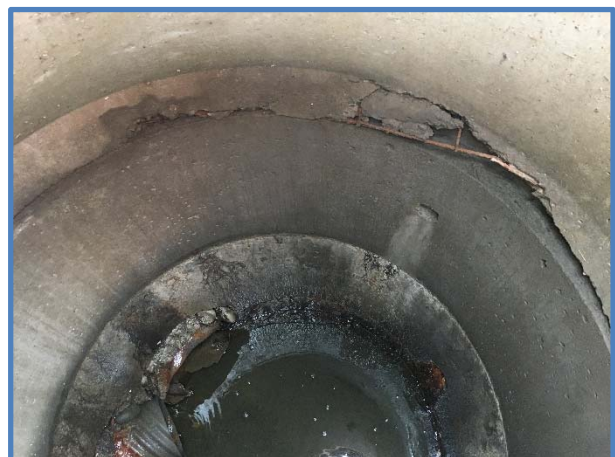
Photo 2 - Cone Damage, Exposed Steel
