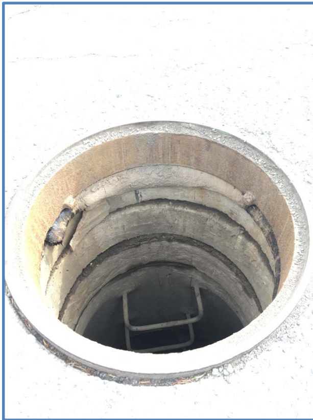
Photo 3 - Frame, Grade Rings & Ladder Rungs
