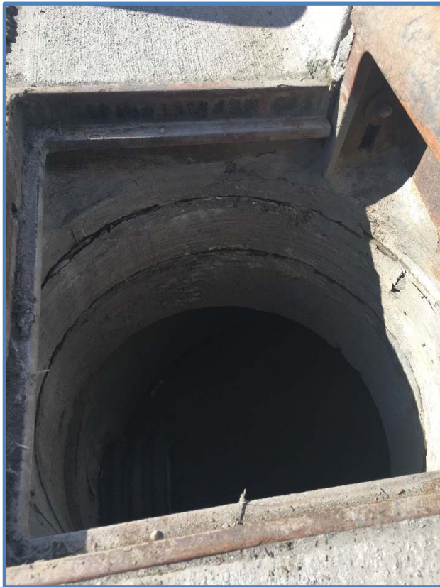
Photo 3 - Frame, Grade Rings & Reducing Slab
