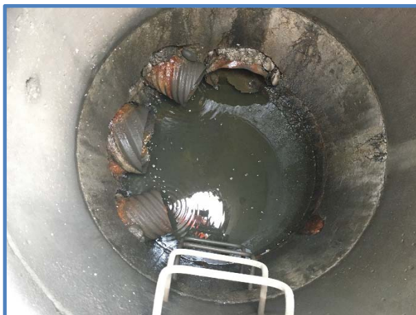
Photo 1 - Inlet & Outlet Pipe Penetrations
