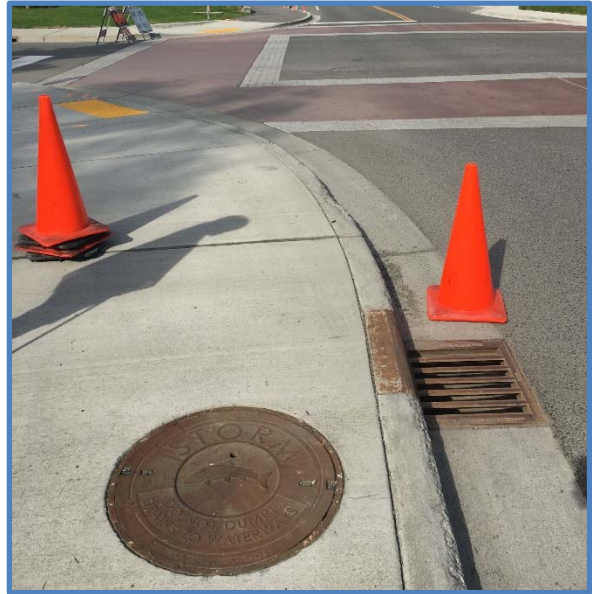
Photo 2 - Type II Catch Basin Manhole / Surrounding Area
