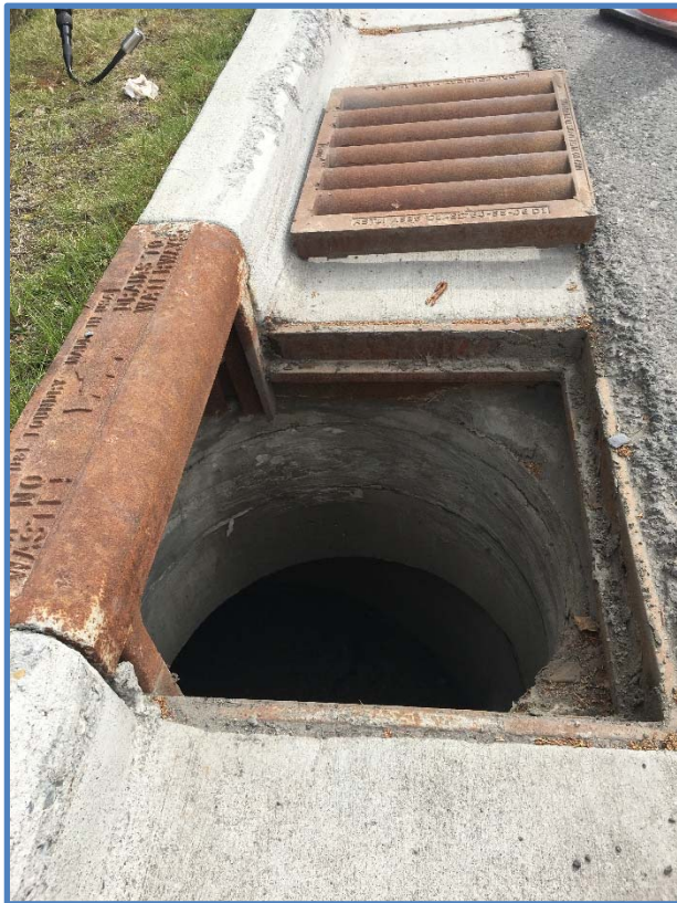
Photo 3 - Frame, Grade Rings & Reducing Slab
