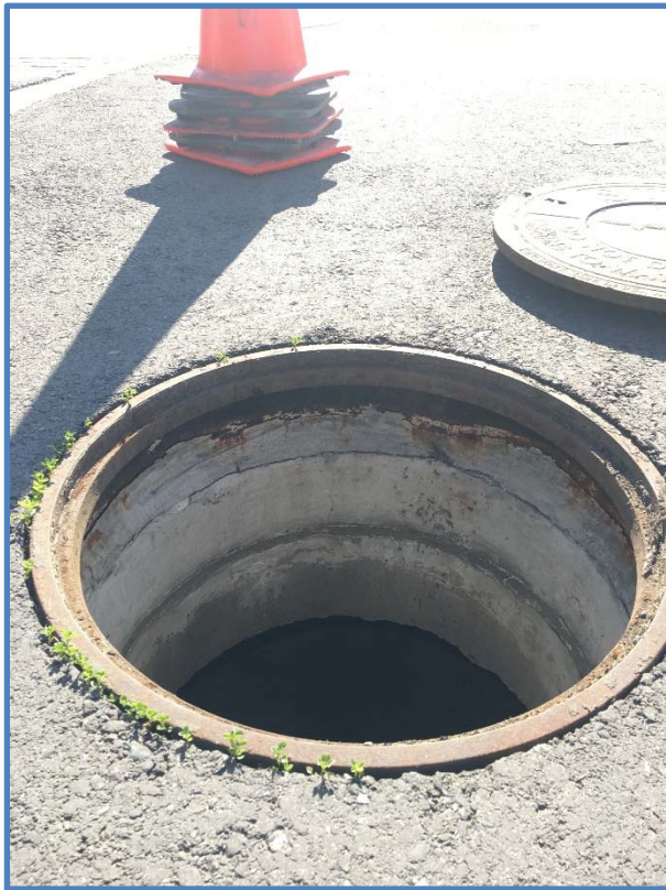
Photo 3 - Frame, Grade Rings & Reducing Slab
