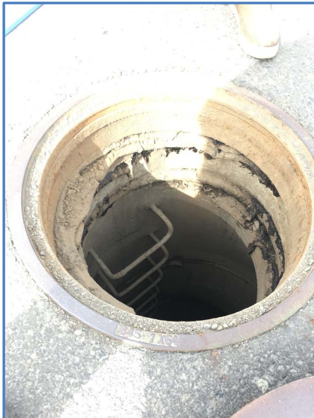
Photo 3 - Frame, Grade Rings & Ladder Rungs
