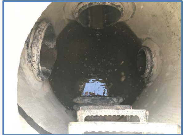
Photo 4 - Inlet & Outlet Pipe Penetrations
