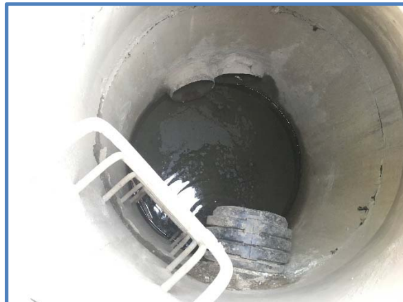
Photo 4 - Inlet & Outlet Pipe Penetrations / End Cap
