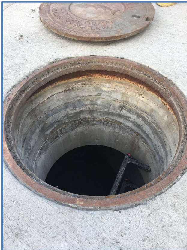
Photo 3 - Frame, Grade Rings & Ladder Rungs
