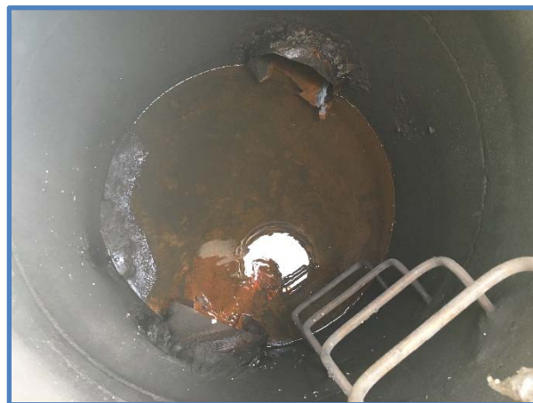
Photo 2 - Inlet & Outlet Pipe Penetrations
