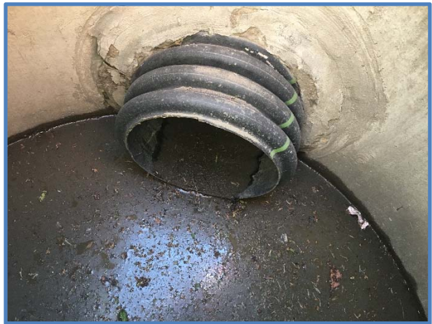
Photo 4 - Outlet Pipe Penetration
