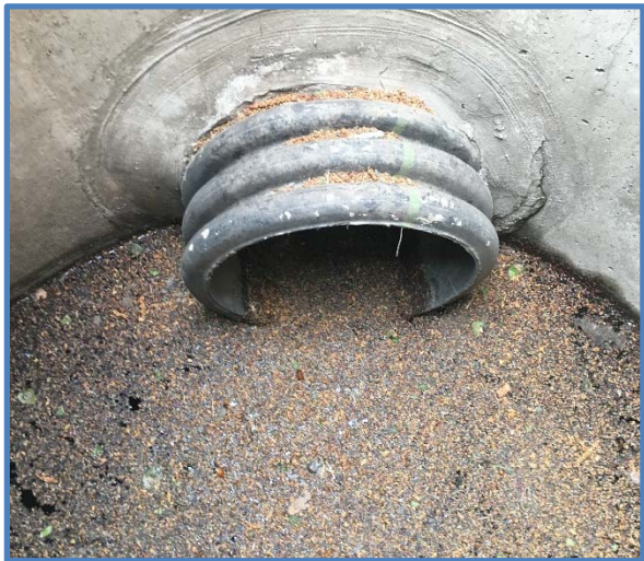
Photo 1 - Outlet Pipe Penetrations
