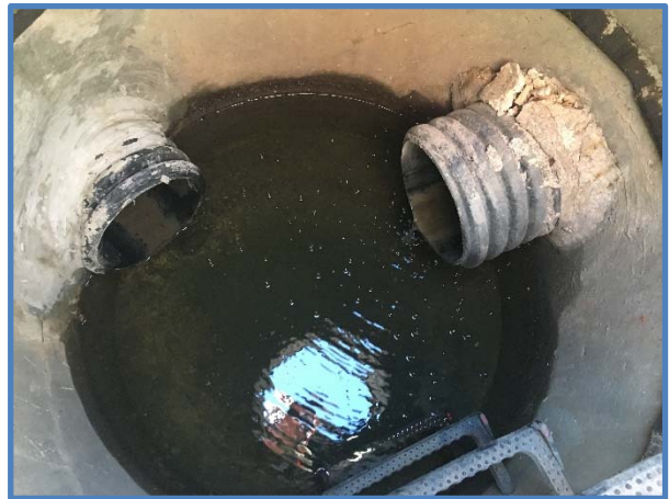
Photo 4 - Inlet & Outlet Pipe Penetrations
