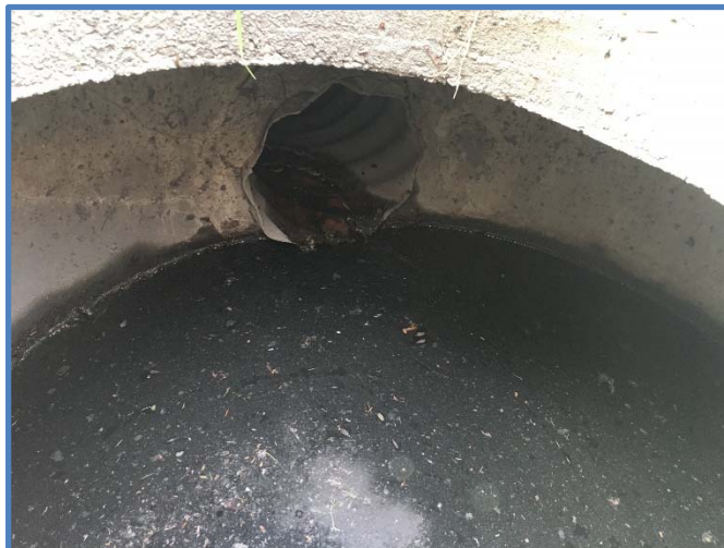
Photo 4 - Outlet Pipe Penetration
