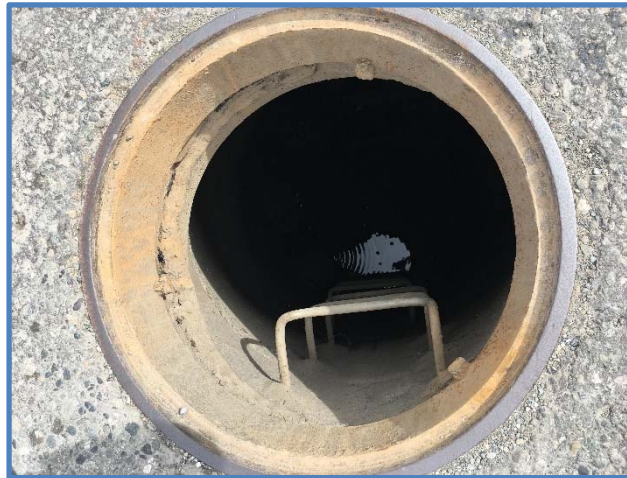
Photo 3 - Frame, Grade Rings & Ladder Rungs
