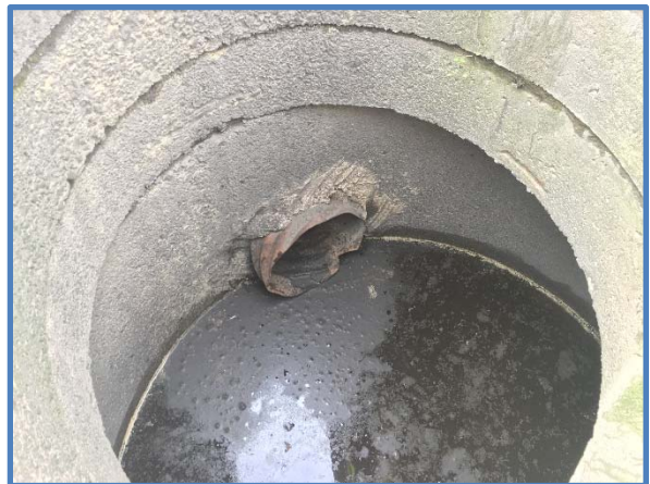
Photo 4 - Outlet Pipe Penetration
