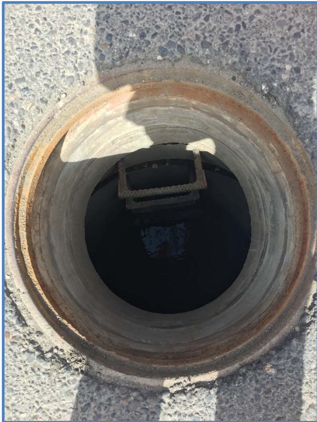
Photo 3 - Frame, Grade Rings & Ladder Rungs
