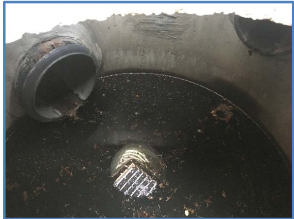
Photo 4 - Inlet & Outlet Pipe Penetrations
