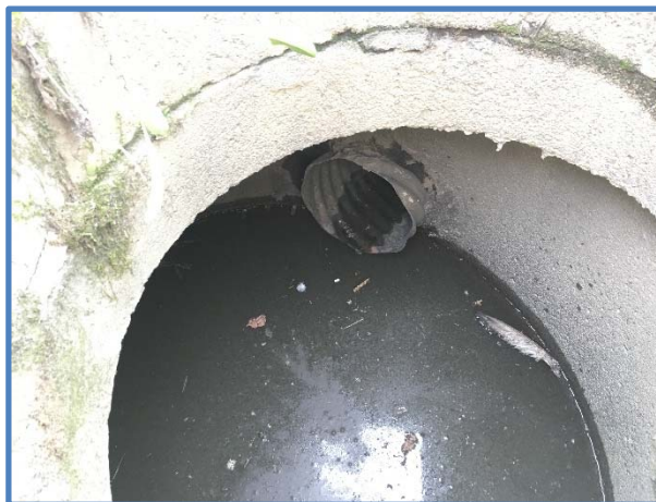
Photo 4 - Outlet Pipe Penetration
