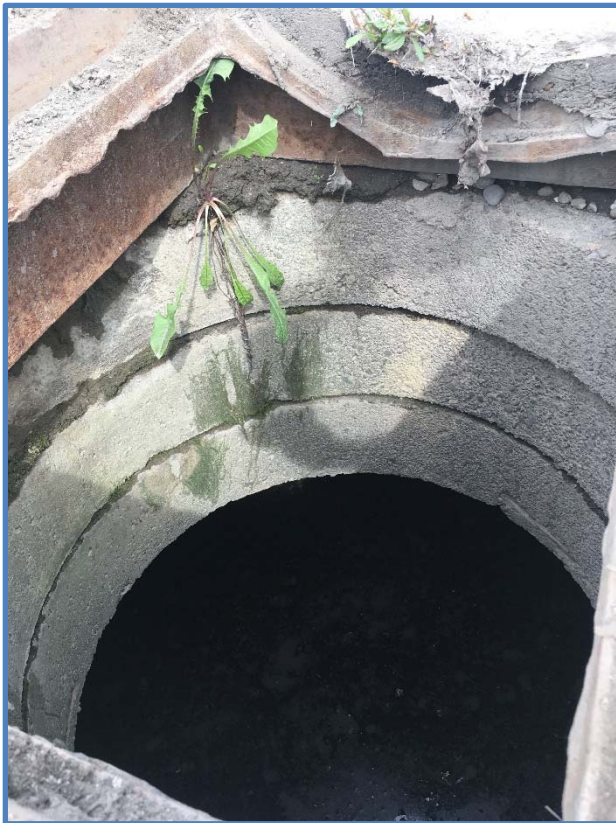
Photo 3 - Frame, Grade Rings & Reducing Slab
