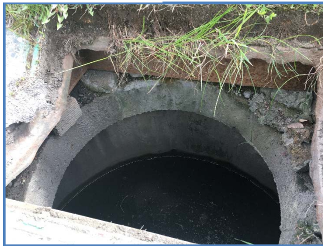
Photo 2 - Frame, Brick Grade Rings & Reducing Slab
