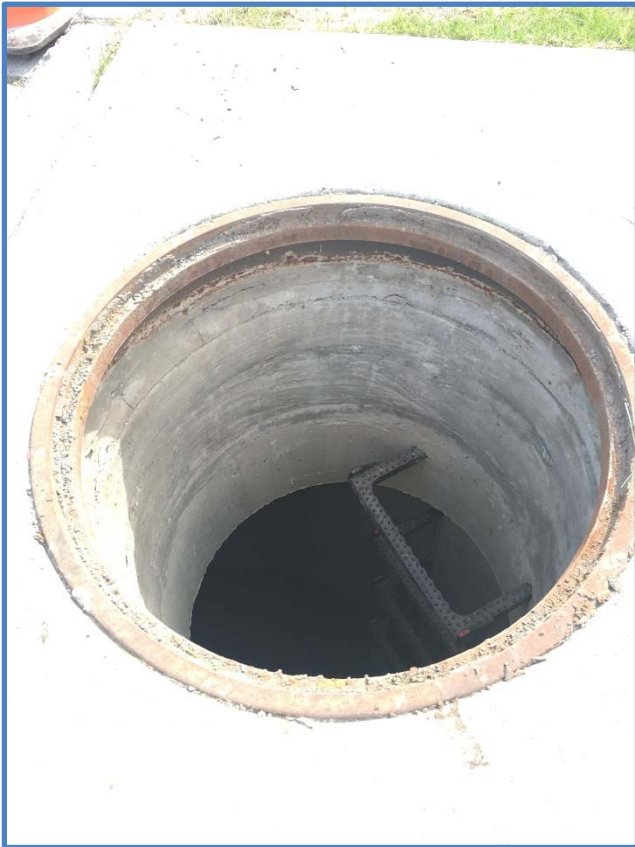
Photo 1 - Frame, Grade Rings & Ladder Rungs
