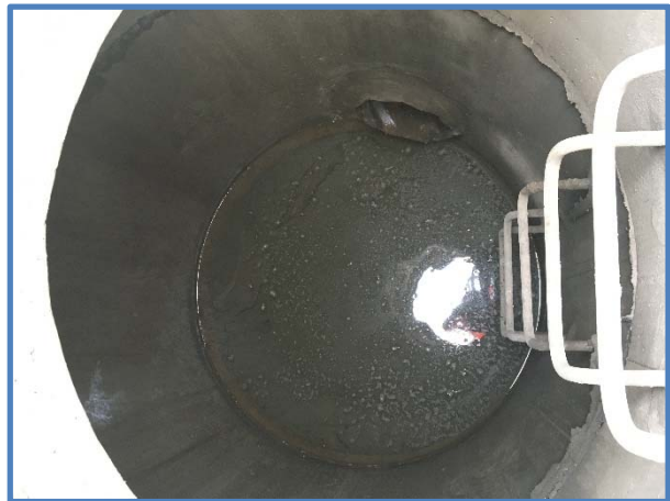
Photo 2 - Outlet Pipe Penetration
