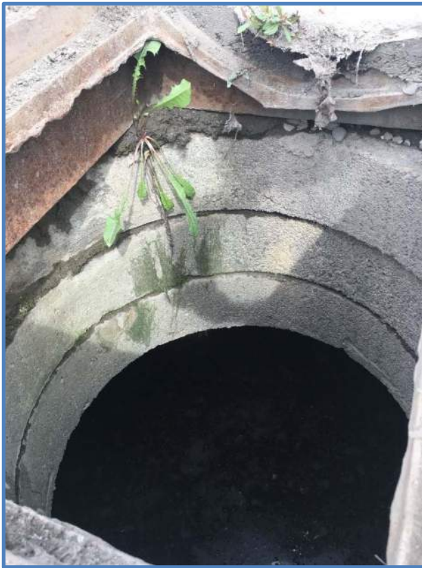
Photo 3 - Frame, Grade Rings & Reducing Slab
