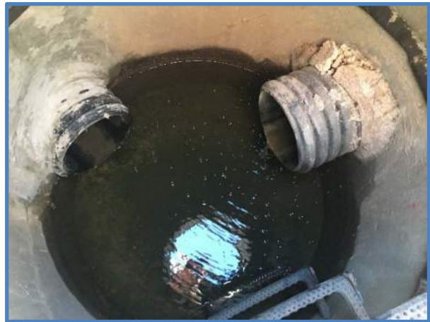
Photo 4 - Inlet & Outlet Pipe Penetrations
