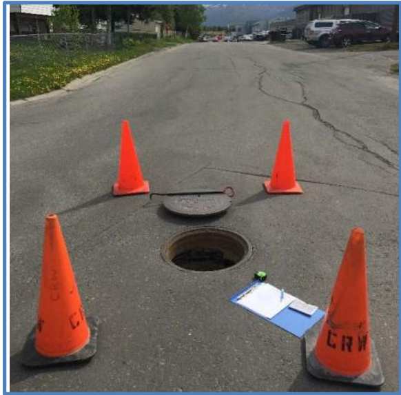
Photo 2 - Manhole / Surrounding Area
