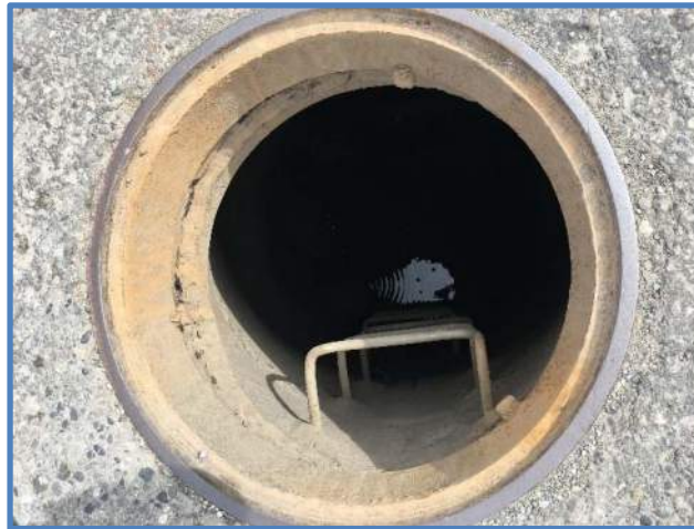
Photo 3 - Frame, Grade Rings & Ladder Rungs
