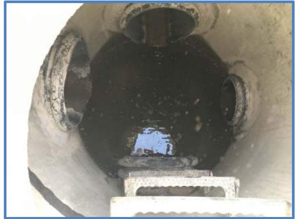
Photo 4 - Inlet & Outlet Pipe Penetrations
