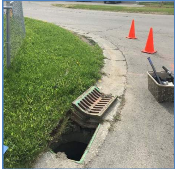
Photo 1 - Curb Inlet / Surrounding Area
