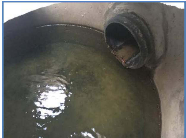
Photo 4 - Outlet Pipe Penetration
