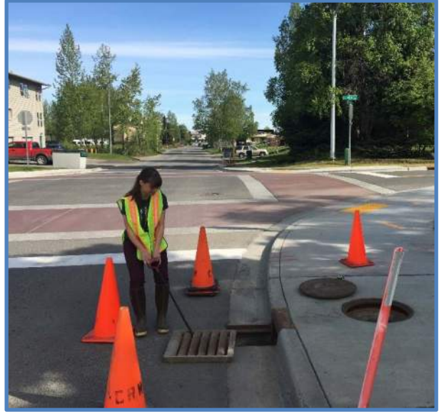
Photo 2 - Type II Catch Basin Manhole / Surrounding Area
