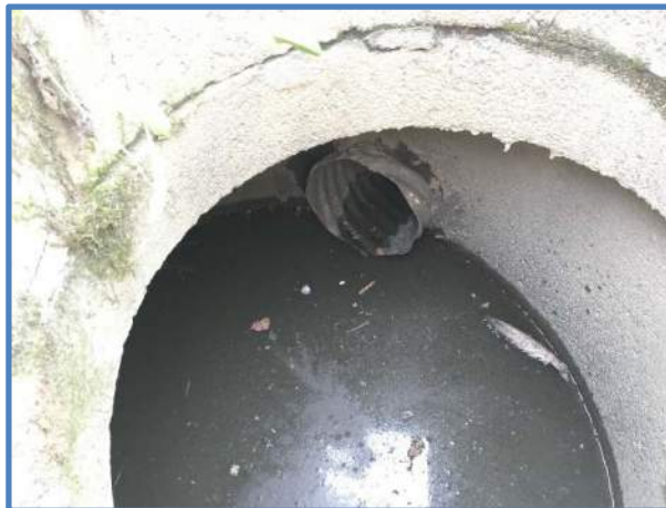
Photo 4 - Outlet Pipe Penetration
