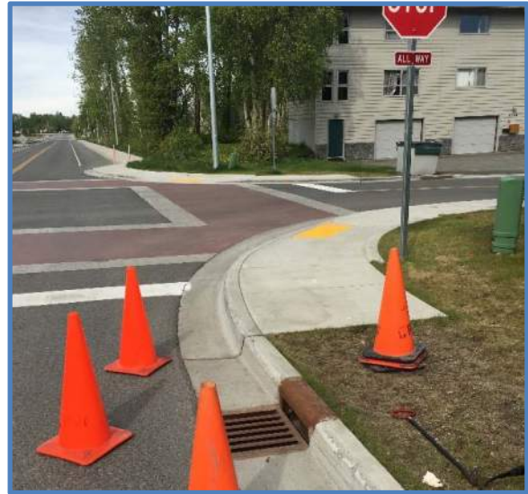
Photo 2 - Curb Inlet / Surrounding Area
