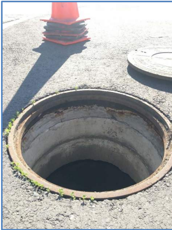
Photo 3 - Frame, Grade Rings & Reducing Slab
