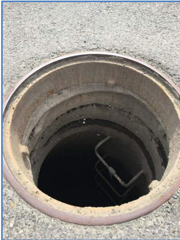
Photo 3 - Frame, Grade Rings & Ladder Rungs
