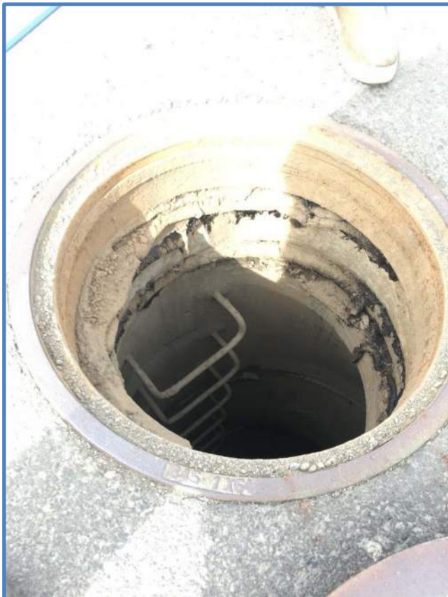
Photo 3 - Frame, Grade Rings & Ladder Rungs
