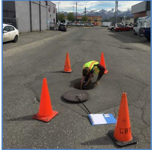
Photo 1 - Manhole / Surrounding Area
