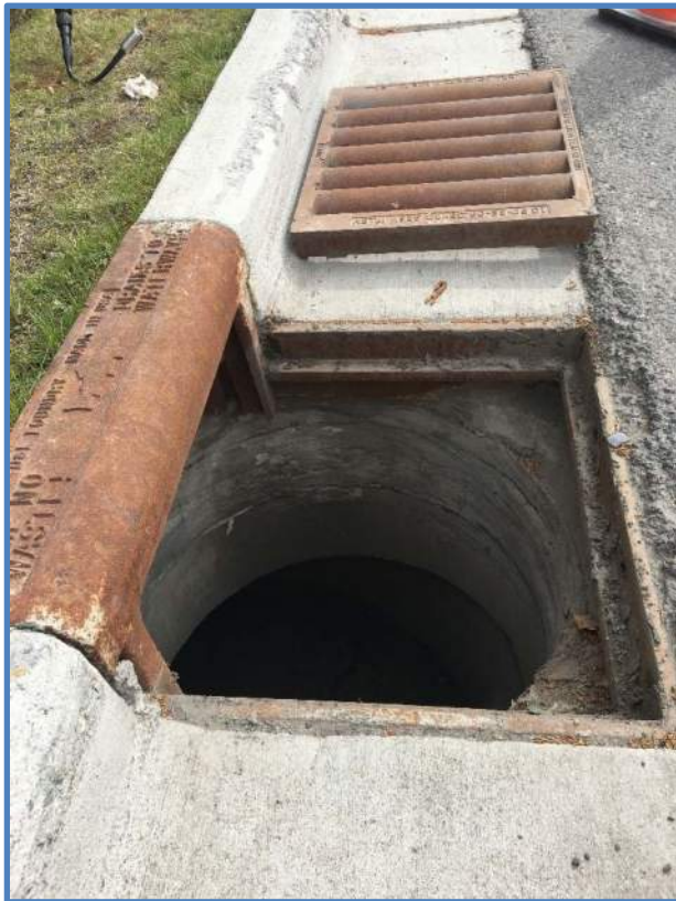
Photo 3 - Frame, Grade Rings & Reducing Slab
