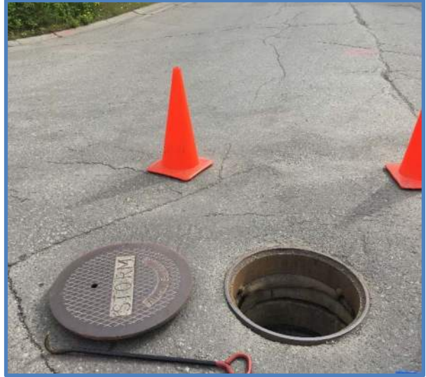
Photo 1 - Manhole / Surrounding Area
