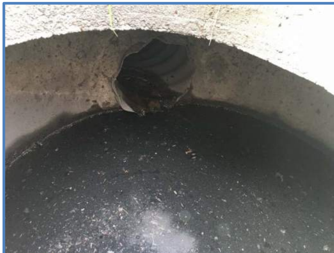
Photo 4 - Outlet Pipe Penetration
