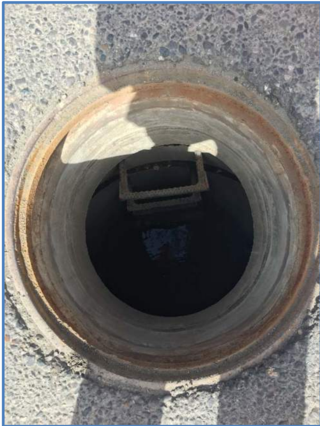
Photo 3 - Frame, Grade Rings & Ladder Rungs
