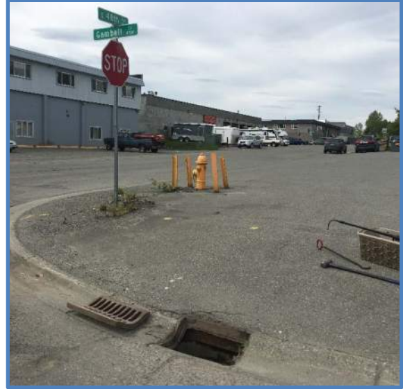
Photo 2 - Curb Inlet / Surrounding Area
