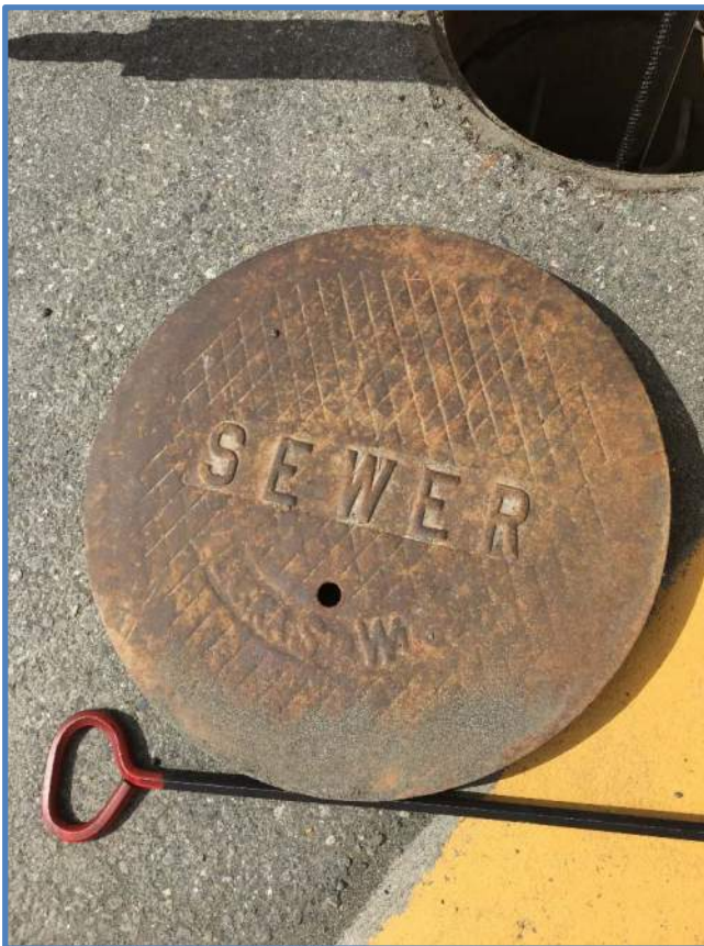
Photo 3 - Sewer Manhole Cover
