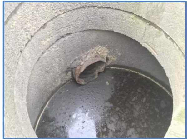
Photo 4 - Outlet Pipe Penetration
