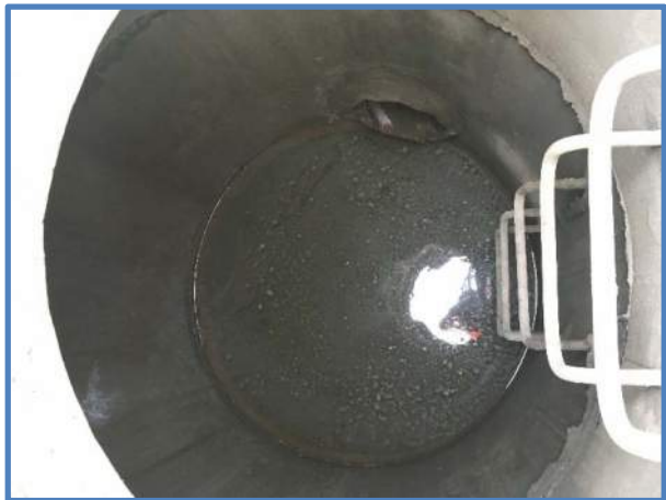
Photo 2 - Outlet Pipe Penetration
