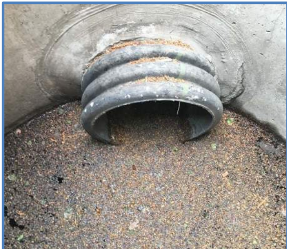
Photo 1 - Outlet Pipe Penetrations
