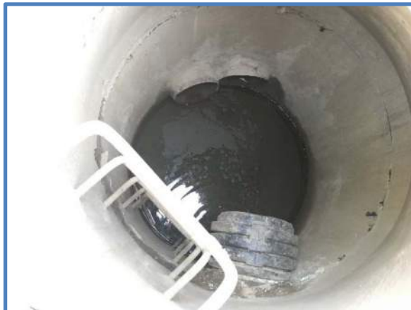
Photo 4 - Inlet & Outlet Pipe Penetrations / End Cap
