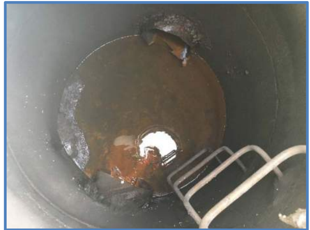
Photo 2 - Inlet & Outlet Pipe Penetrations
