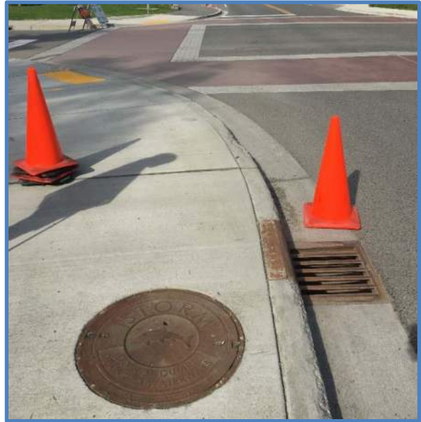
Photo 2 - Type II Catch Basin Manhole / Surrounding Area
