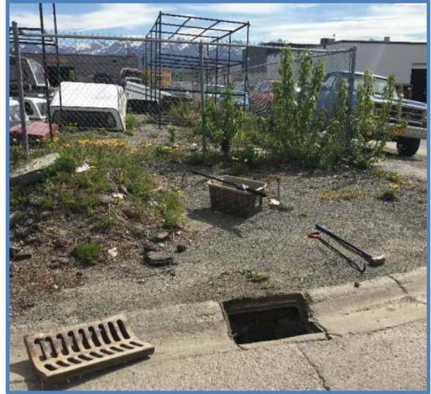
Photo 2 - Curb Inlet / Surrounding Area
