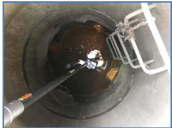
Photo 4 - Inlet & Outlet Pipe Penetrations
