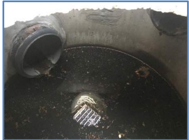
Photo 4 - Inlet & Outlet Pipe Penetrations
