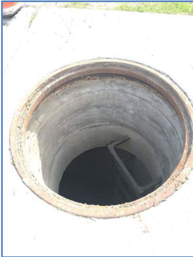
Photo 1 - Frame, Grade Rings & Ladder Rungs
