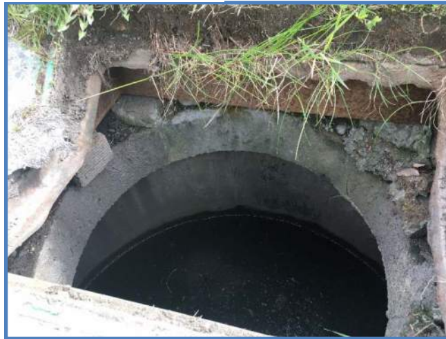
Photo 2 - Frame, Brick Grade Rings & Reducing Slab
