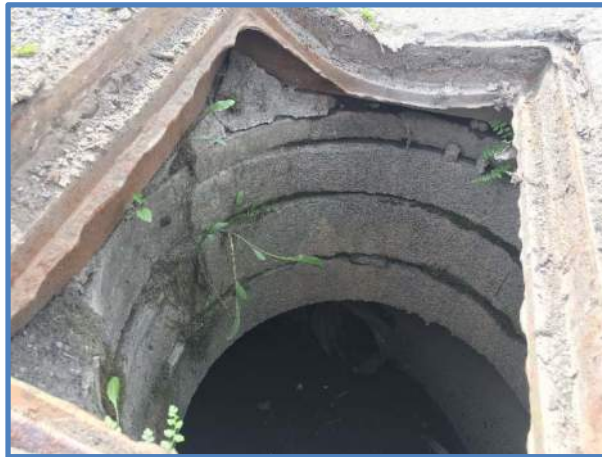
Photo 3 - Frame, Grade Rings & Reducing Slab
