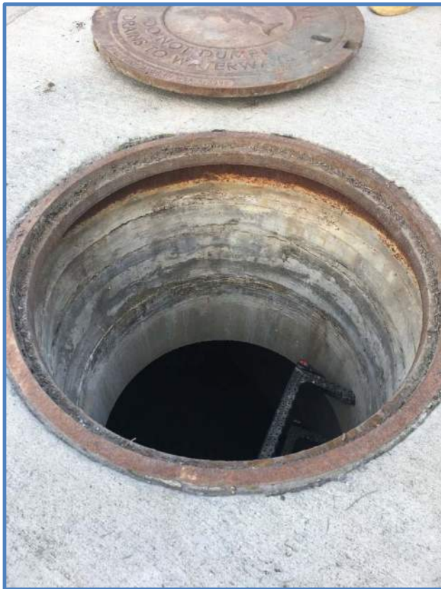
Photo 3 - Frame, Grade Rings & Ladder Rungs
