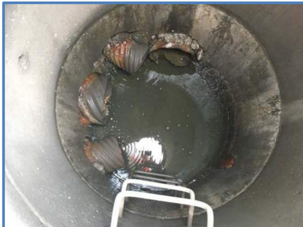
Photo 1 - Inlet & Outlet Pipe Penetrations
